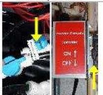
Close "TO flush valve". Turn RO controller switch to ON position.
