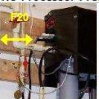
Close RO processor inlet valve F20
