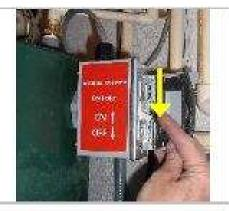
Turn RO controller switch to OFF position.
