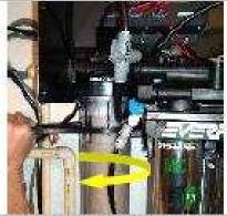
Rotate clear sump left with sump wrench. Rinse sump with mild soap solution.
